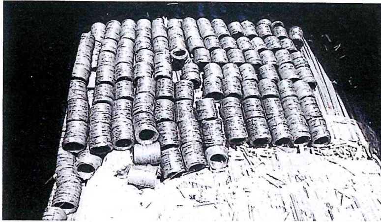
✓ Plastic sheets used to segregate the rebar from the WRIC
