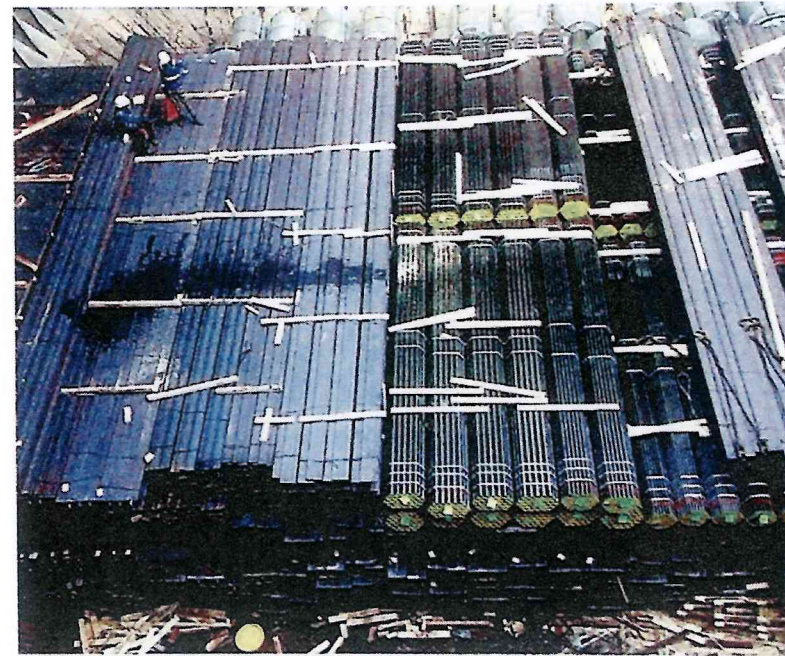
✔ Bundled pipes loaded over structural steel
