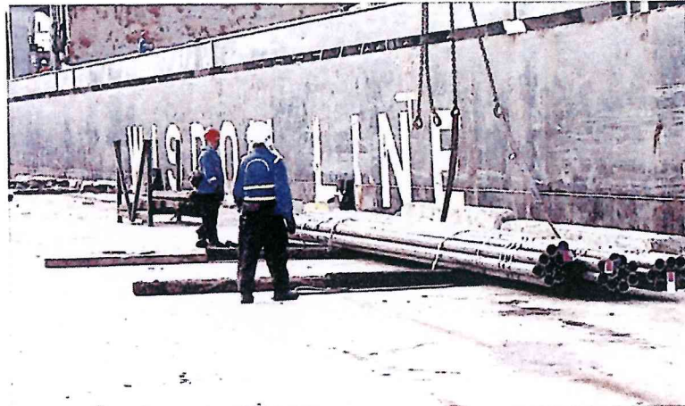
Discharging pipes with a single basket sling and placing the pipes on the quay
