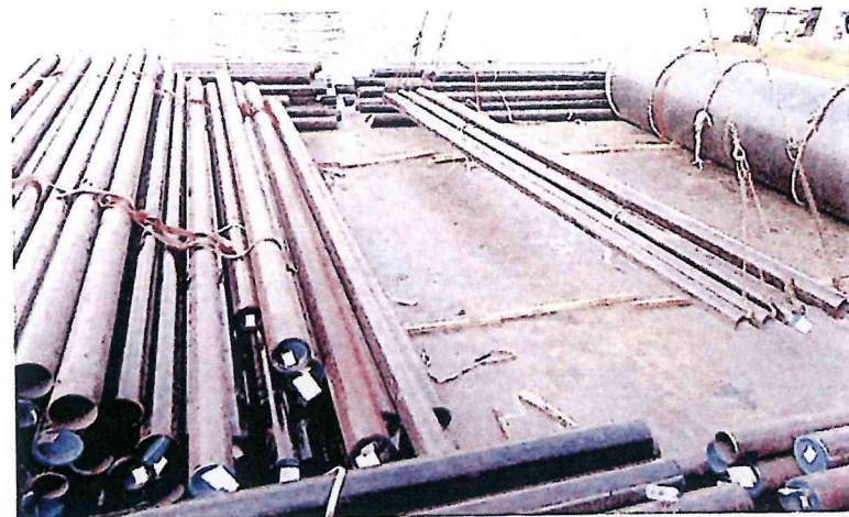
The pipes discharged with hooks to barges. The pipes should be pre-slung
