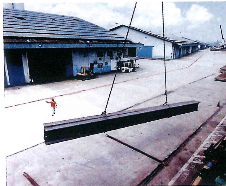
An application of the two-leg chain choke hitch around I-beams
