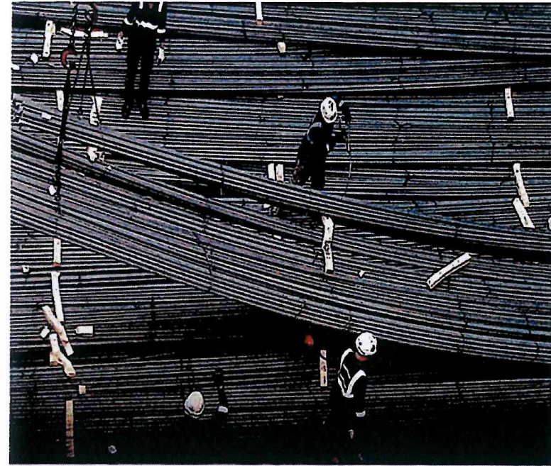
✓ Tip-lifting technique used for discharging rebar
