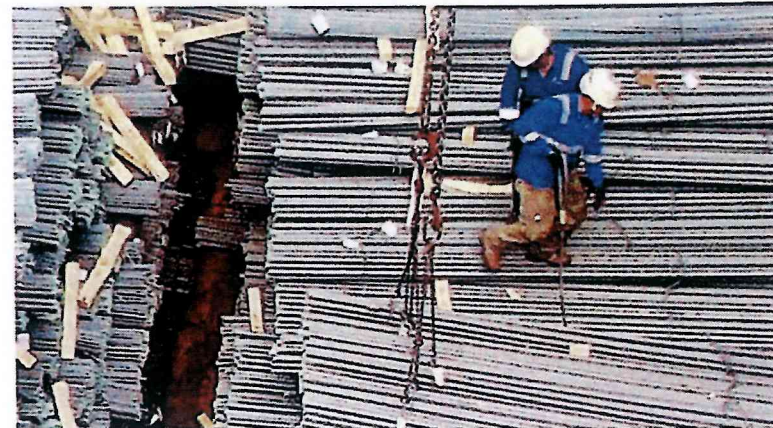
✓ Tip-lifting from the end of the rebar bundles
