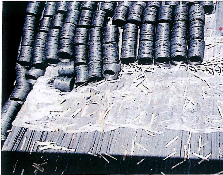
WRIC loaded on top of rebar, segregated with plastic sheets
