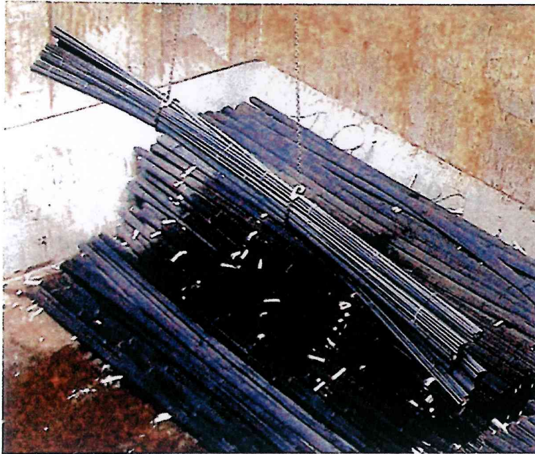
✓ An application of the two-leg chain choke hitch around the bundles
