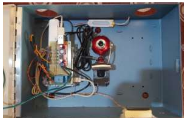
Fig. 4 Installation of the Access control system.
