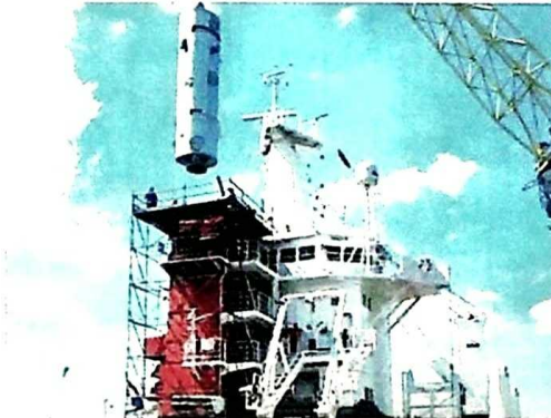
Retrofitting scrubber on an existing ship
