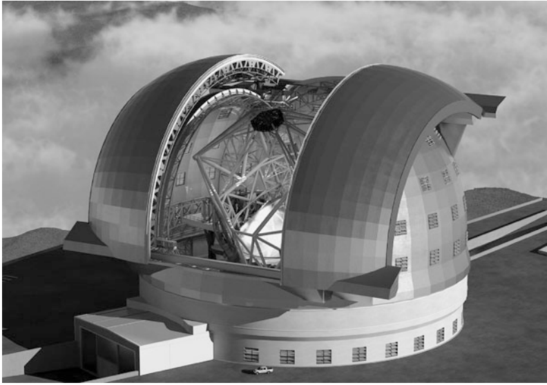
Fig. 3.21 In order to observe objects essentially fainter than nowadays the size of the objective must be increased considerably. The European Southern Observatory ESO started to make plans for a 100 metre OWL telescope (Overwhelmingly Large telescope), but when the price turned out to be “astronomical” the size has been reduced
