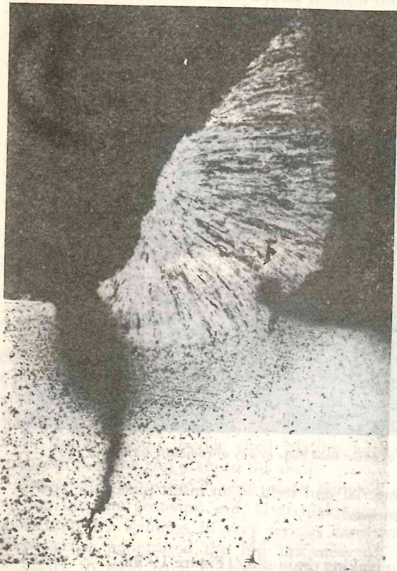
Figure 19.4 A photomicrograph of a section taken through a defective connection of the end plate to a furnace. An open crack is clearly visible in the furnace plate at the toe of the sealing weld. Lack of penetration at the endplate connection is also evident
