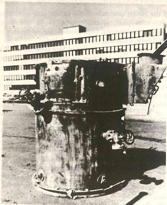
Figure 19.14 Remains of vertical boiler after steam drum had torn off through overpressure
