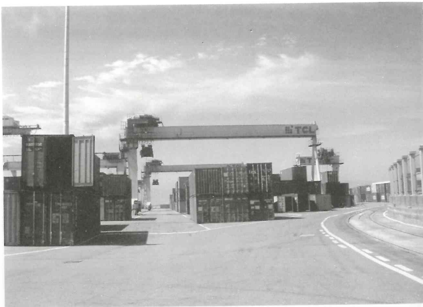
Fig. 8.30 Tracked, terminal stacking gantry cranes operate through the Lisbon container terminal. Rail and road transport having access to the container park.
