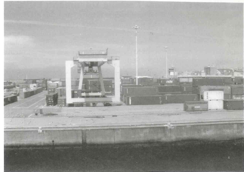
Fig. 8.31 Walkways, road paths and track rails for gantry cranes seen alongside the berth, opposite the terminal stacking gantries. Container avenues lying parallel to the ships berth.
