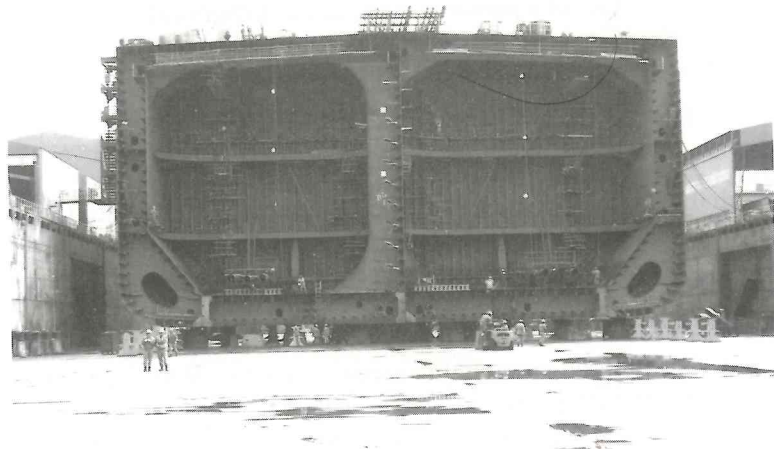
Fig. 5.5 Athwartships cross-section of the modern double-hull tanker seen at a late construction stage prior to assembly.
