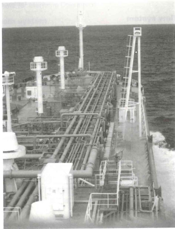
Fig. 5.9 Tanker deck arrangement. Typical example of the pipeline (fore deck) arrangement of a medium size oil tanker seen in the sea-going environment.
