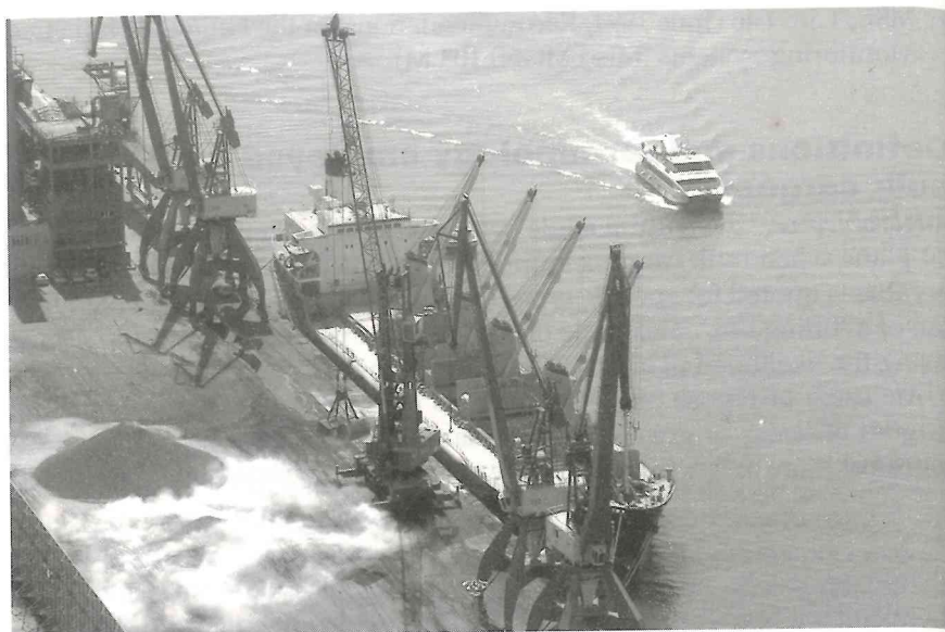
Fig. 4.2 An overhead view of a general cargo vessel engaged in the discharge of concentrates by means of a free-standing crane using a mechanical grab. The ship's own deck cranes are turned outboard to allow easy access for the shoreside crane operation.
